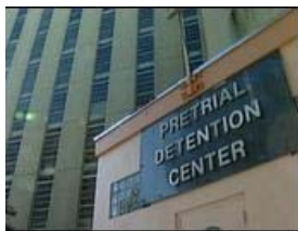
The Miami-Dade Pre-Trial Detention Facility, where mentally ill inmates are held.
